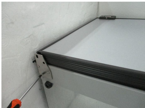
1. Unscrew the 2 hinges (6 screws)
