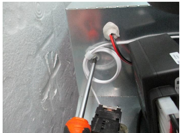
4. Unscrew the plastic support
