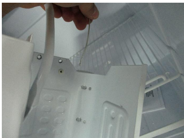
5. Remove the thermostat bulb
