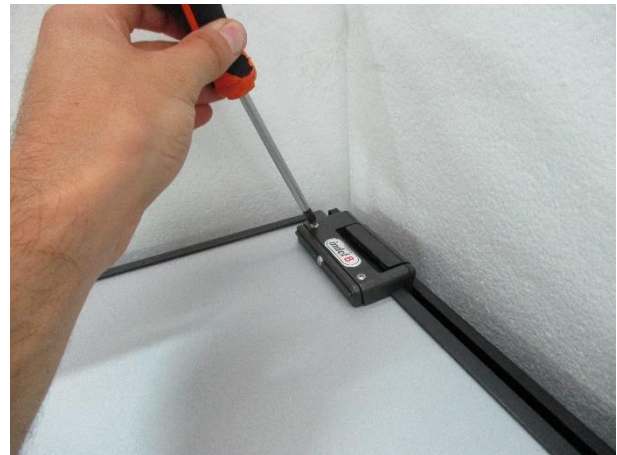
4. Unscrew the handle (3 bolts)
