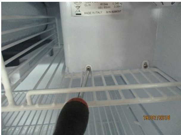
7. Unscrew the balcony (2 screws)
