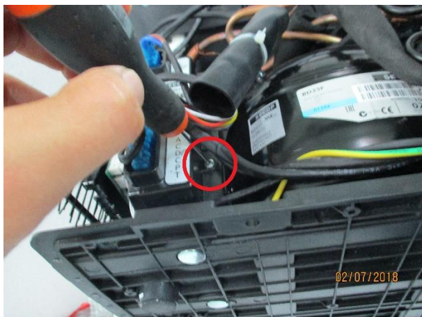
5. Unscrew the bolt in figure
